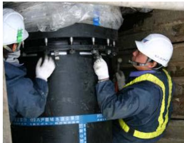
DIP with seismic flexible joint
