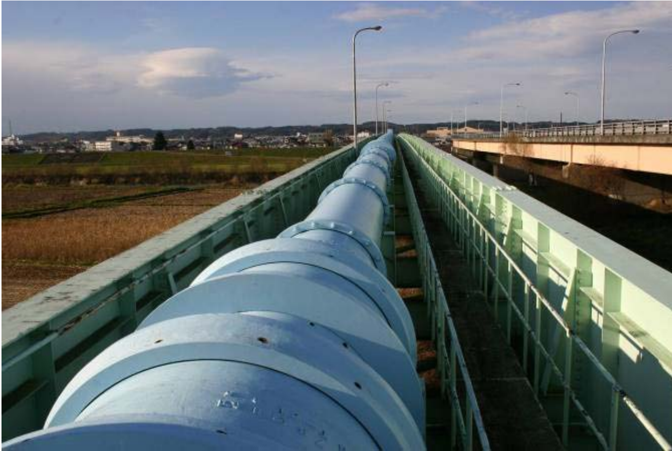
DIP with seismic flexible joint ( \phi 1,000\text{mm} ) : completed in 1978
