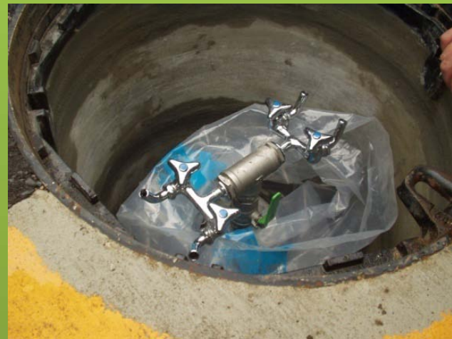
Underground hydrant
