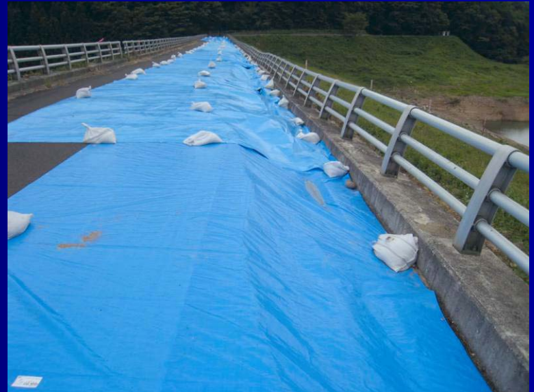
Protect cracks from water intrusion (from GEER, Japan 2008 EQ)
