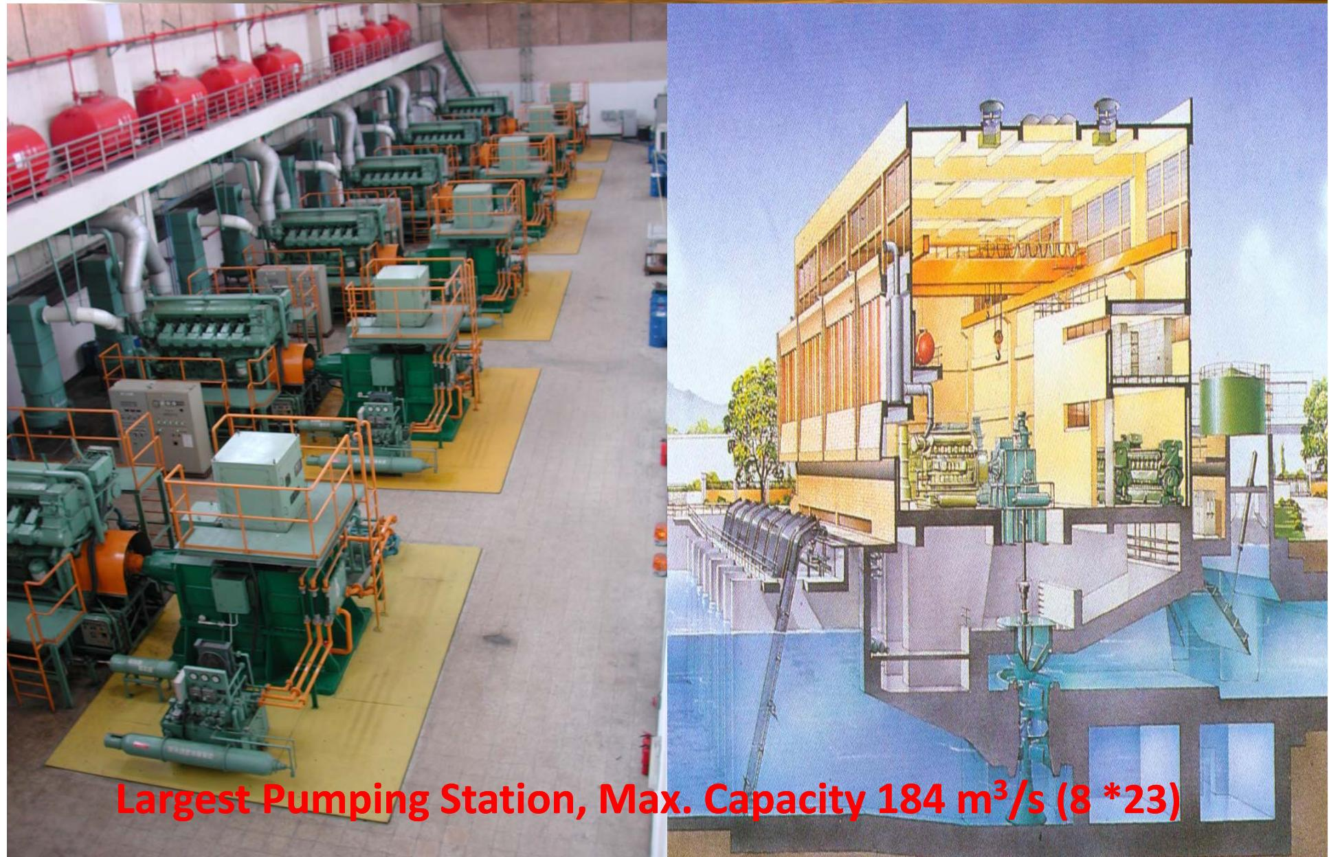
Largest Pumping Station, Max. Capacity  $184 \text{ m}^3/\text{s}$  (8 \*23)
