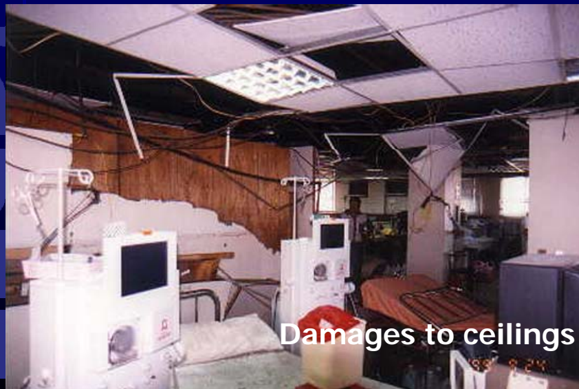
■ Fall-off of air condition outlet
