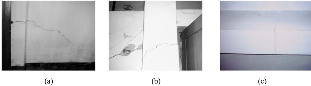
Figure 3: Patterns of damages of structural elements (a) Typical wall (b) Typical column (c) Typical beam
