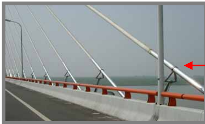
Figure 32 MR is used in Ton-Tin Lake Bridge in China
