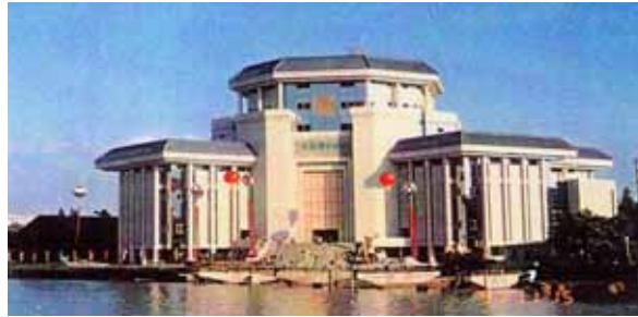
Figure 8: RC frame-shear 13 stories museum with story isolation
