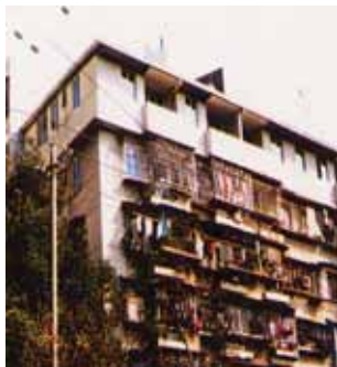
Figure 25: Adding Stories of Top of Building
