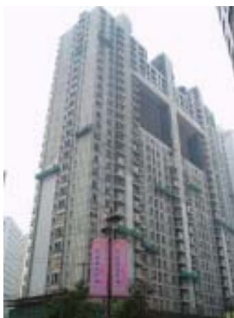
Figure 12. Construction of the irregular building
